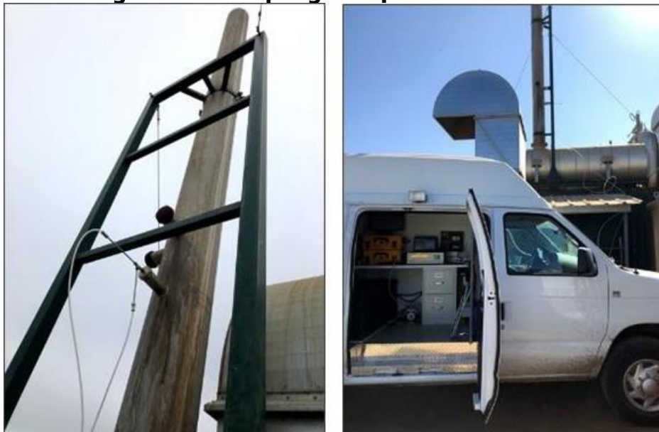
Figure 16: Sampling Setup at CHP Exhaust
